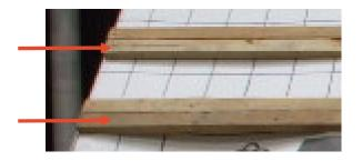
The purpose of this double/extra batten is to support the top of the natural slate.
