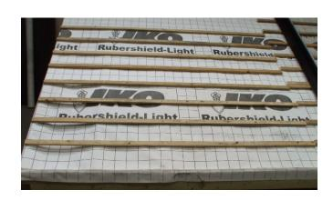
Fit double battens on the batten above any natural slate.
